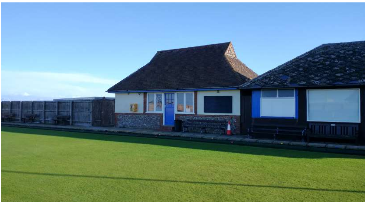
To remain and be refurbished
